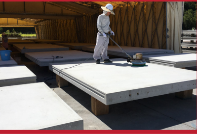
Polishing and cleaning precast concrete slabs. So much trust.
